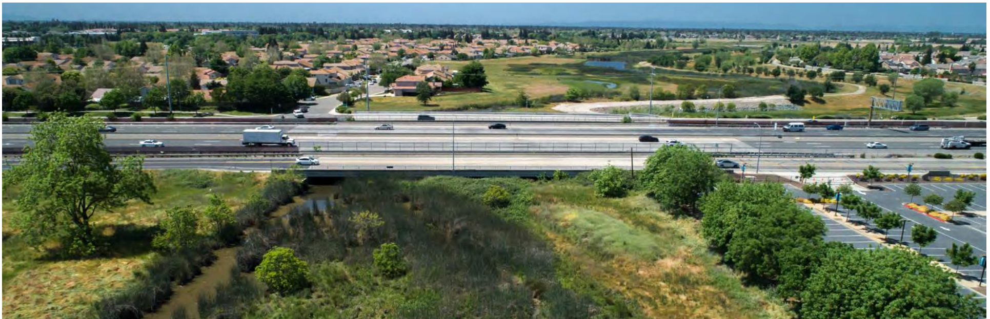
State Route 99 bridge over Elk Grove Creek.
